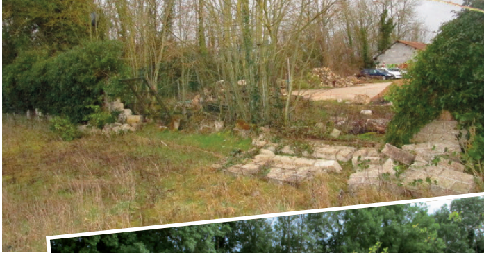
Mur clôture services techniques
